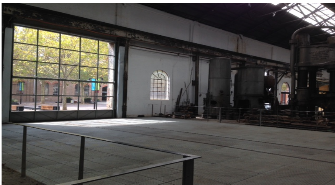
Figure 16: Photograph from site visit to Eveleigh Locomotive workshop, June 2014
