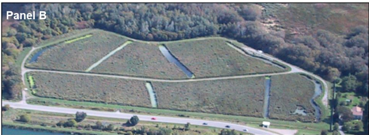
Figure 1-2: Cross section schematic (Panel A) and top view photo (Panel B) of a typical surface flow constructed wetland (SFCW). Adapted from CH2M Hill (2014).
