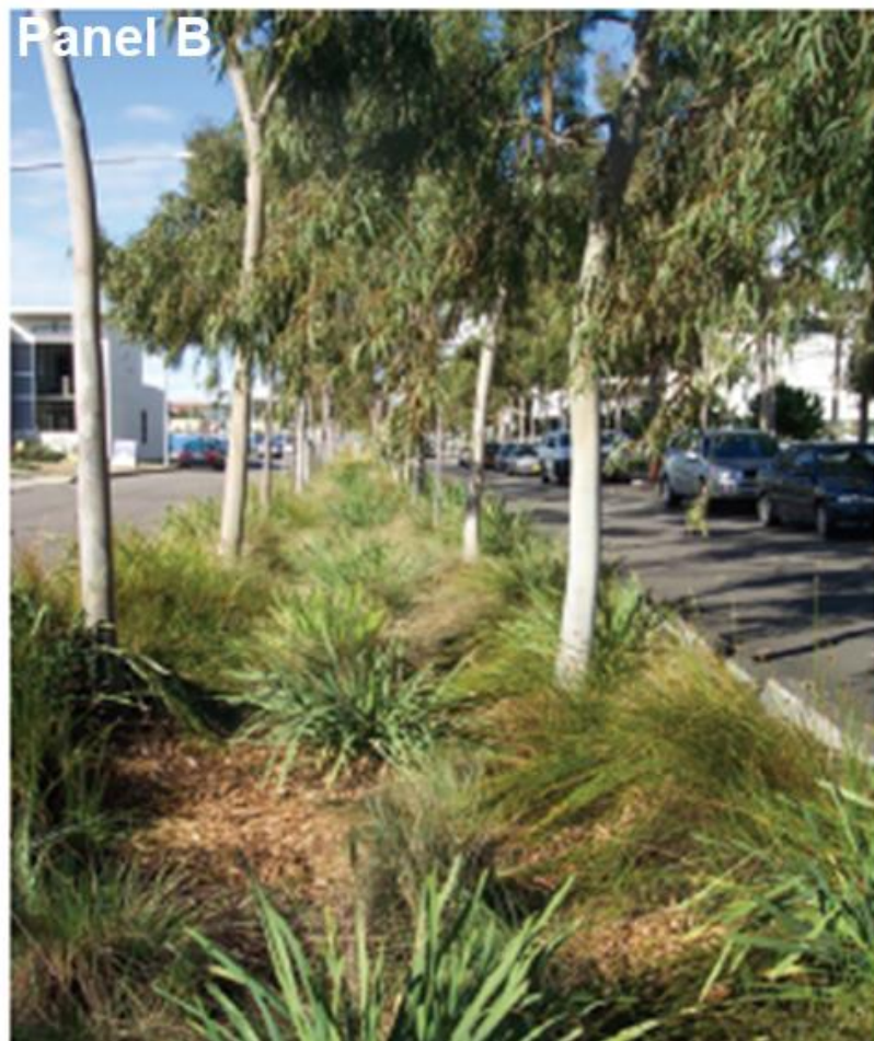
Figure 1-3: Cross section schematic (Panel A) and top view photo (Panel B) of a typical stormwater biofilter. Adapted from Macnamara & Derry (2017) (A) and Zinger et al. (2007) (B).
