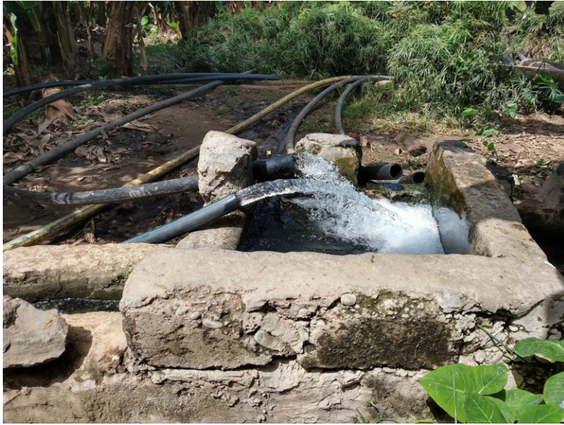
Picture 4:2 Water being pumped into temporary reservoirs. Rocha Lama, Cabo Verde.
