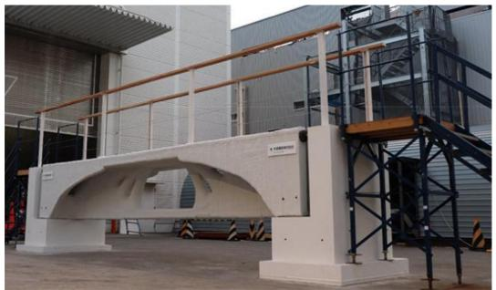
Figure 3.8 3D printed pre-stressed concrete bridge by Taisei Corporation [57].
