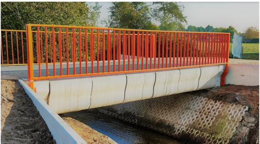
Figure 3.5 Bicycle bridge in Gemert made by BAM Infra and TU/e [51].
