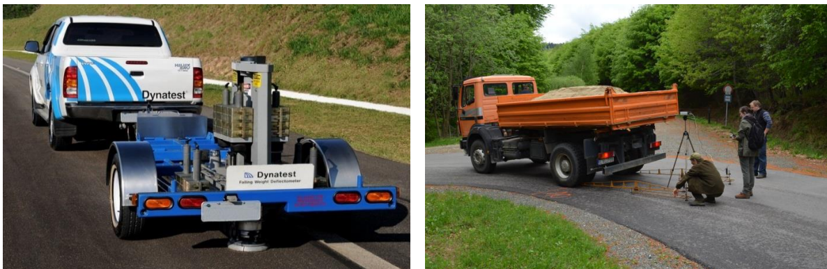
Figure 1. Falling Weight Deflectometer (left) and Improved Benkelman Beam Apparatus (right) in action.
