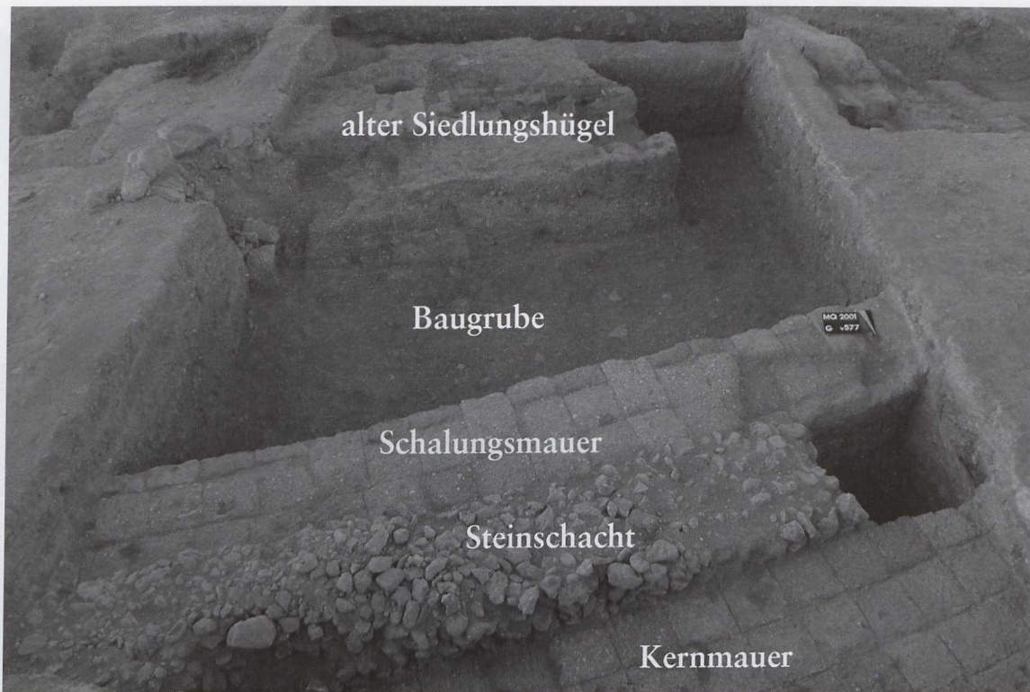
Abb. 4 Fundamentgrube in Raum B (Foto: Monika Perkovic).
