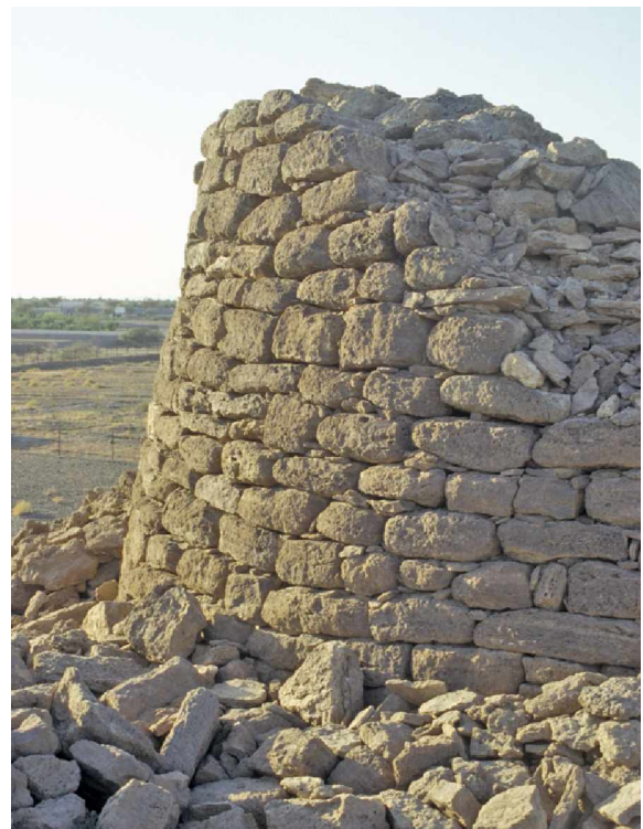
Fig. 25. Masonry of one of the towers at Ḥalban.
