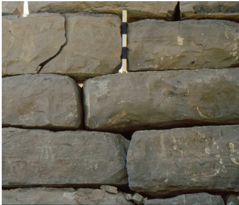
Fig. 20. The large blocks from tower A at Yānqūl were flaked and picked (left of the scale).
