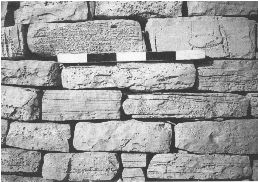
Fig. 17. The dressed stones of Shi2 show traces of flaking their outer edges.
