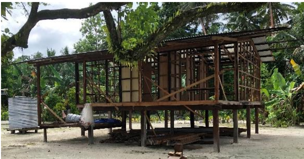
Figure 7.4 A permanent house (with water tank) being constructed with BDM earnings.
