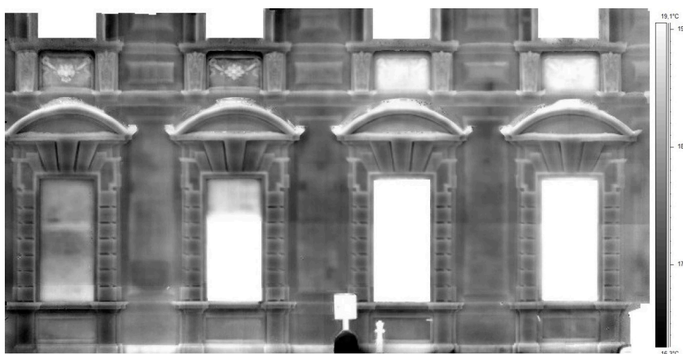
Figure 13. Thermal orthophoto-mosaic produced with FLIR 660SC imagery.
