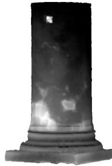
Figure 14. View of final 3D thermal model of a column's base, where the position of restoration materials can be observed.
