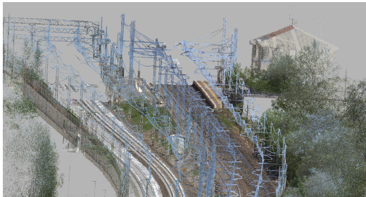
Figure 1. Example of train mobile mapping point cloud acquired in proximity of a station.
