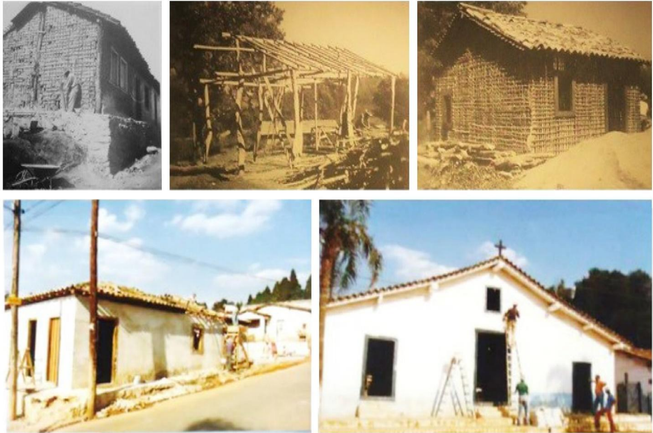
Figure 5. Different stages of renovation of the Apericube Village.
