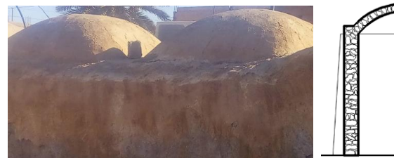
Figure 3. (a) Domes of a building in Guemar. (b) Section of wall and dome.
