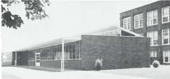
INDUSTRIAL ARTS BUILDING
