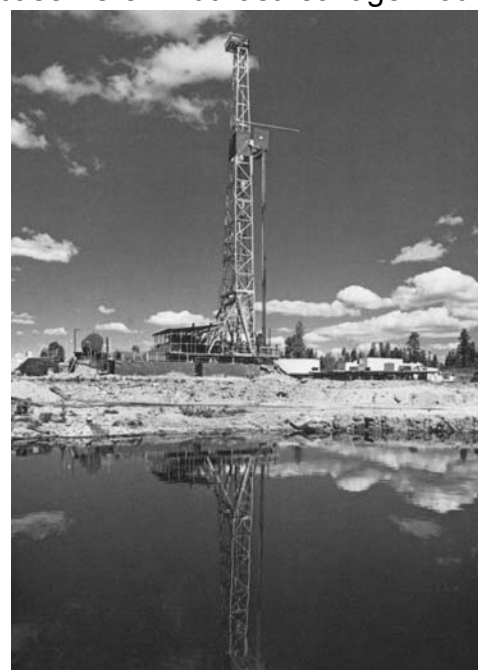
Figure 2 Drilling rig at Fenton Hill, NM. Photo by Los Alamos National Laboratory.
