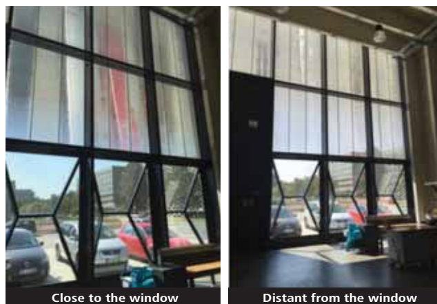
Figure 4: Interior projection of daylight by a prismatic glazing at TU Darmstadt, Darmstadt, Germany.
