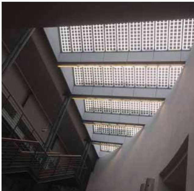
Figure 2: Atrium with a semi-transparent photovoltaic glazed roof at the Fraunhofer Institute for Solar Energy Systems, Freiburg, Germany.
