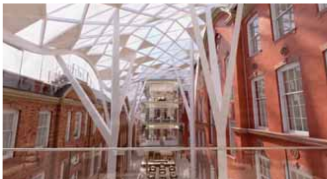
Figure 7: An atrium retrofitted between existing buildings at Sheffield University, UK. (Anon, 2020).
