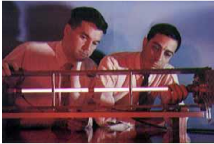
Fig.10 Herriot and Javan with the helium-neon optical gas maser [36].
