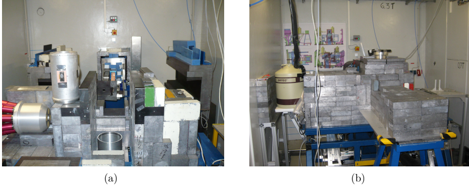
Figure 3.6: (a) A picture taken during the installation of the PGAA facility at FRM II, with the sample chamber in the middle lower part, the interchangeable ends of the beam guide on the middle upper part and a BGO detector at the detector position to the right [70]. (b) A picture of the completed setup.
