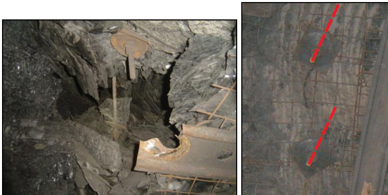
Fig. 6. Close setting of parallel roof bolts
