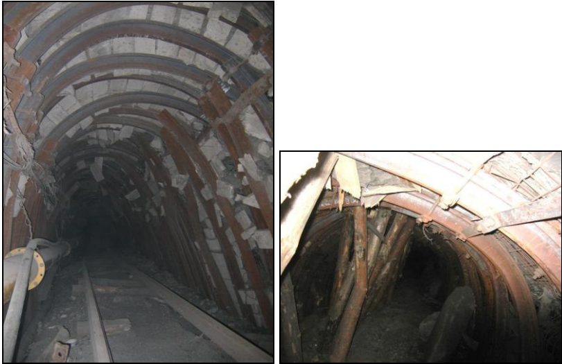
Fig. 1. Roadways with the frame supports
