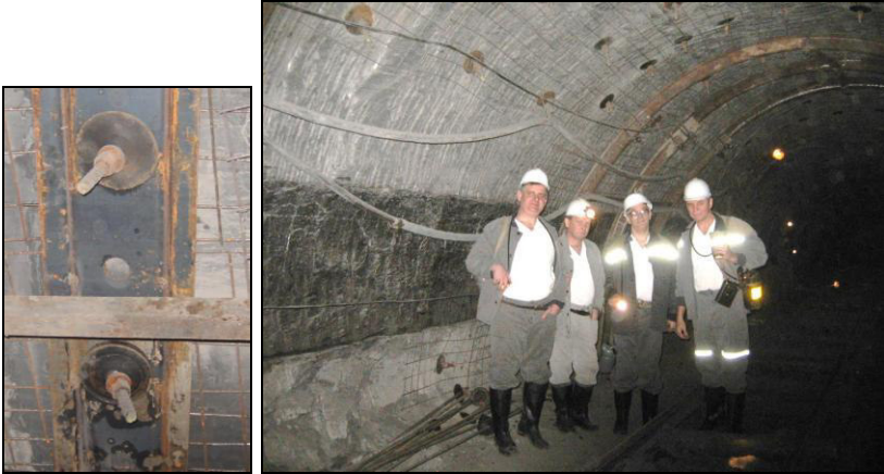
Fig. 8. Testing of the roof-bolt constructions in coal mains
