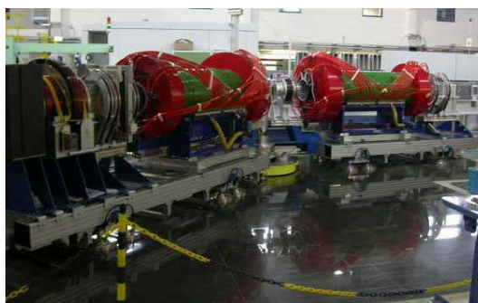
FIG. 2: The NSE spectrometer during installation in the neutron guide hall.
