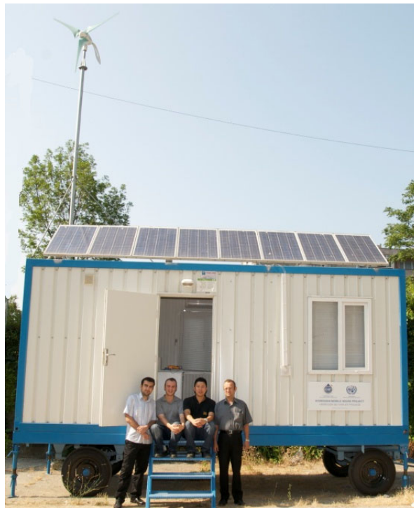
Figure 3: The mobile house with hybrid power system.
