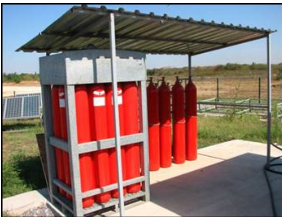
Figure 5a: Hydrogen cylinders.
