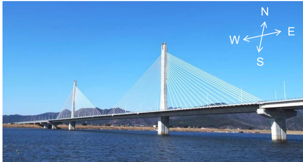
Figure 5. Hwamyung cable-stayed bridge
