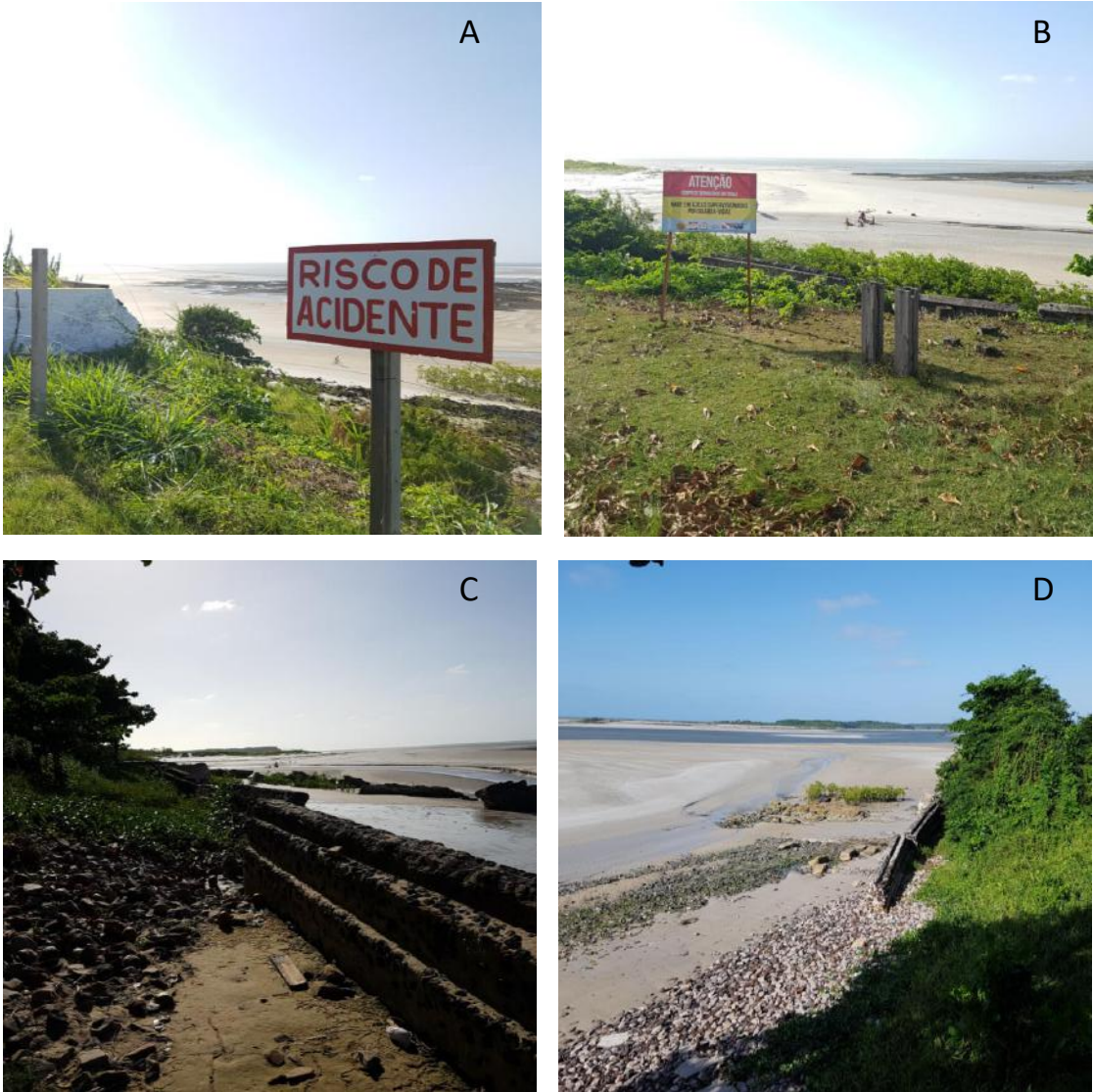
Figure 1.3: Photographs from the isolated area of the cliff and warning signs (photos A and B) and from the remaining of the seawall (photos C and D).
