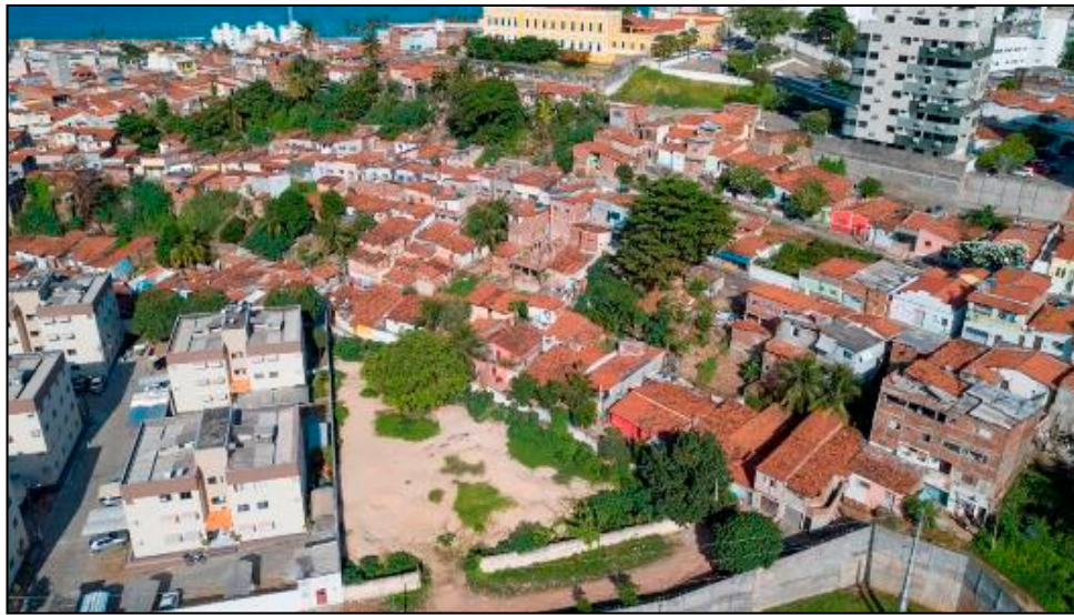
Figure 14. Construction of homes halfway up the slope.
