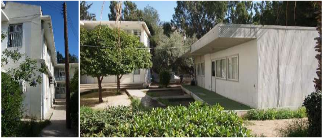
Il. 4- 20/DMS & Il. 4- 21/DMS The main entrance at the southwest façade of the school's initial building @ Author, March 2018
