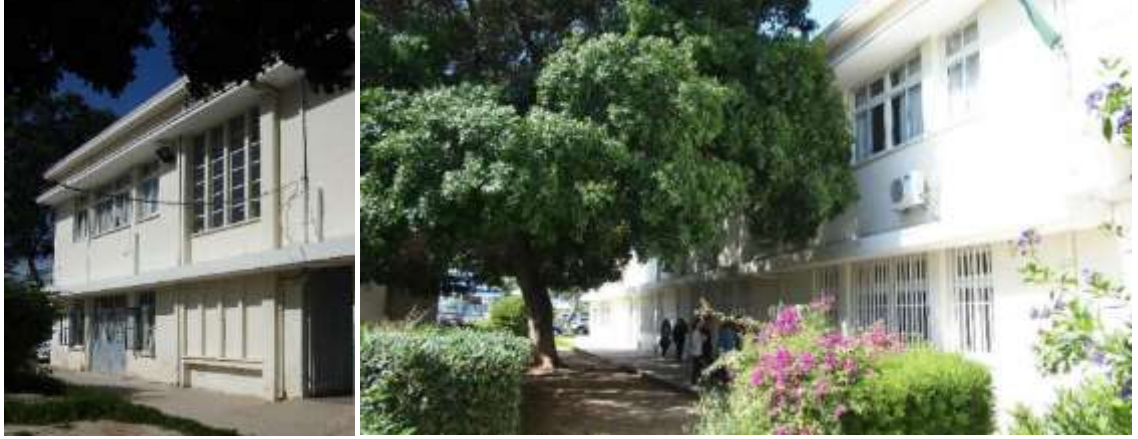
Il. 4- 18/DMS & Il. 4- 19/DMS The westernmost area of the southwest façade of the school's initial building @ Author, March 2018
