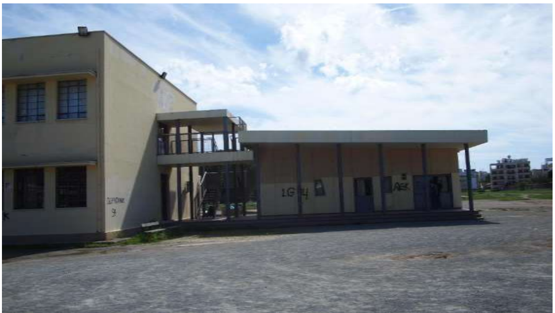
Il. 4- 18/AGHS Recent school extension, west of the south wing, view towards the east @ Author, March 2018
