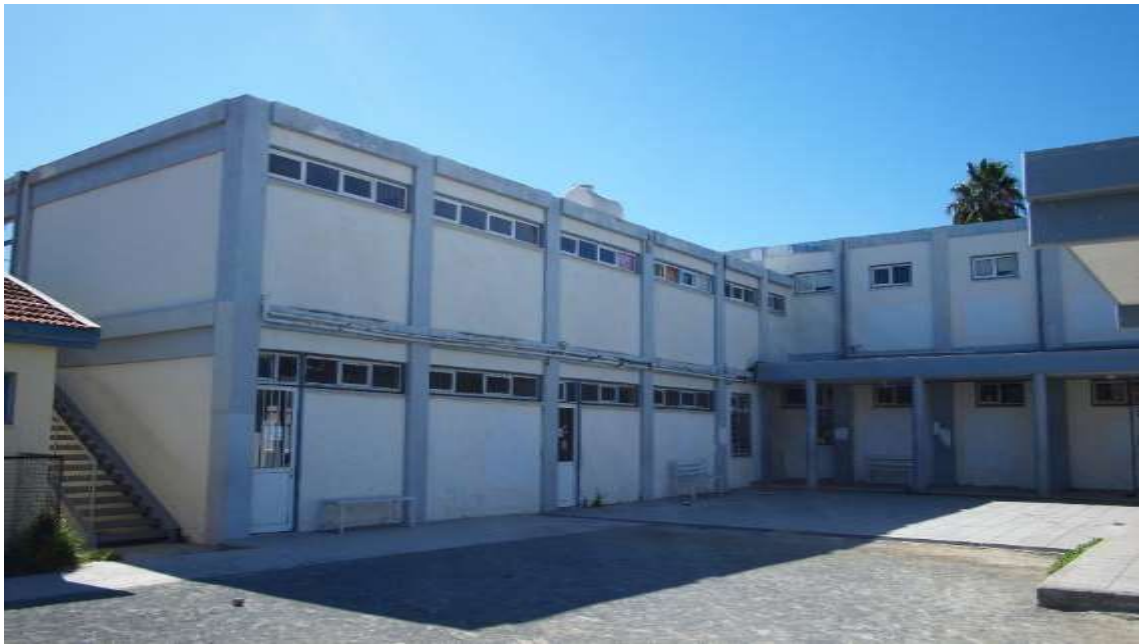
Il. 4- 28/PES North and west façade of the school, view towards the east @ Author, April 2018
