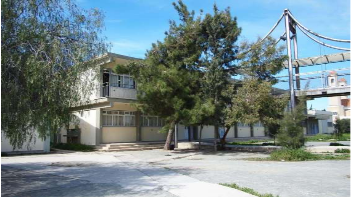
Il. 4- 19/AGHS The recently added western wing of the school, view towards the northwest @ Author, March 2018
