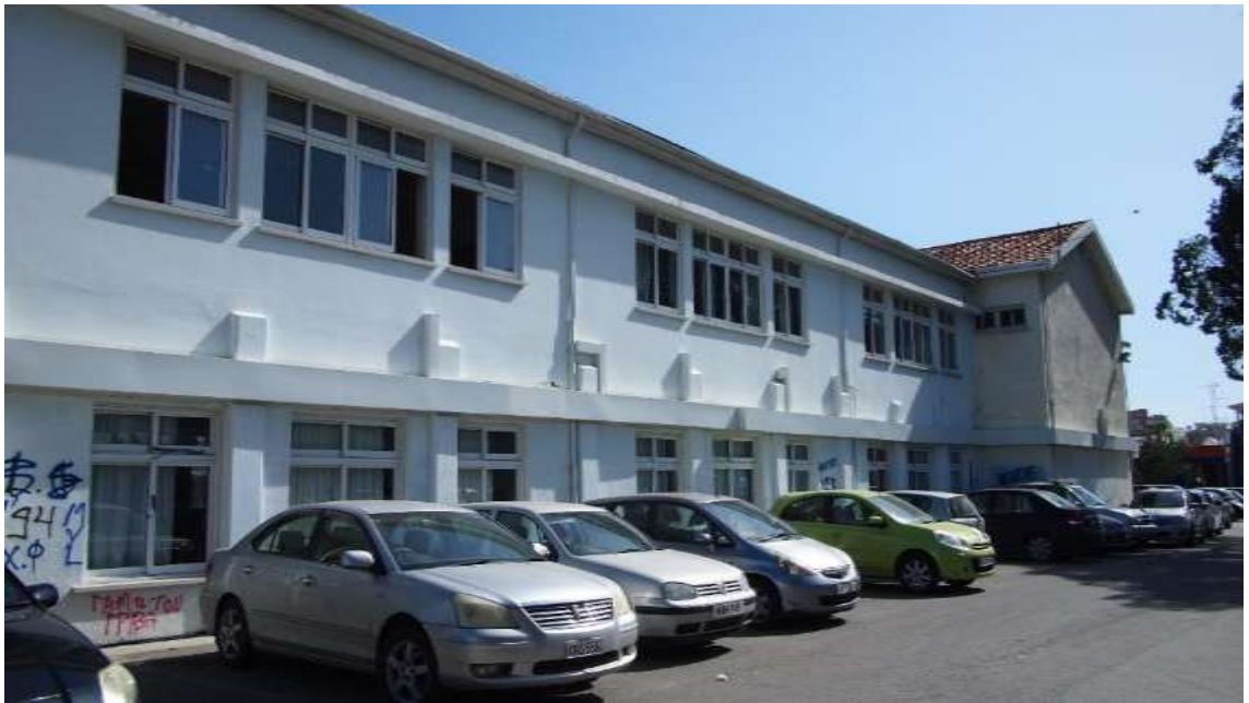
Il. 4- 22/DMS Northwest façade of the school @ Author, March 2018
