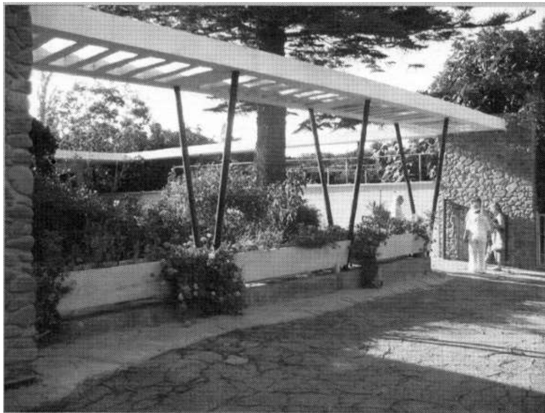
Il. 1- 18 The Sömek House and Clinic, Nicosia @ Retrieved from https://issuu.com/docomomo.cyprus/docs/_importantbuildingsdocomomoc_18_04 [accessed 15 January 2019]
