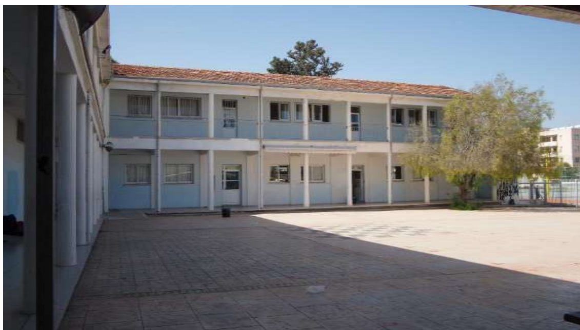
Il. 4- 25/DMS The southeast façade of the northwest wing of the school @ Author, March 2018
