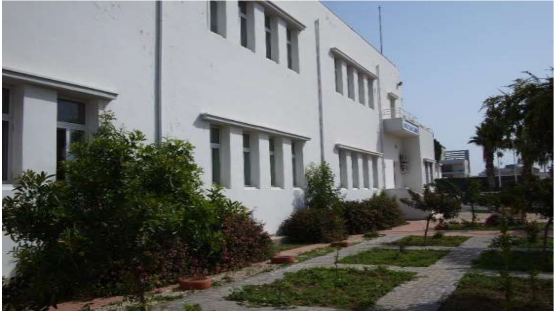
Il. 4- 15/AGES South façade of the school's initial building @ Author, March 2018
