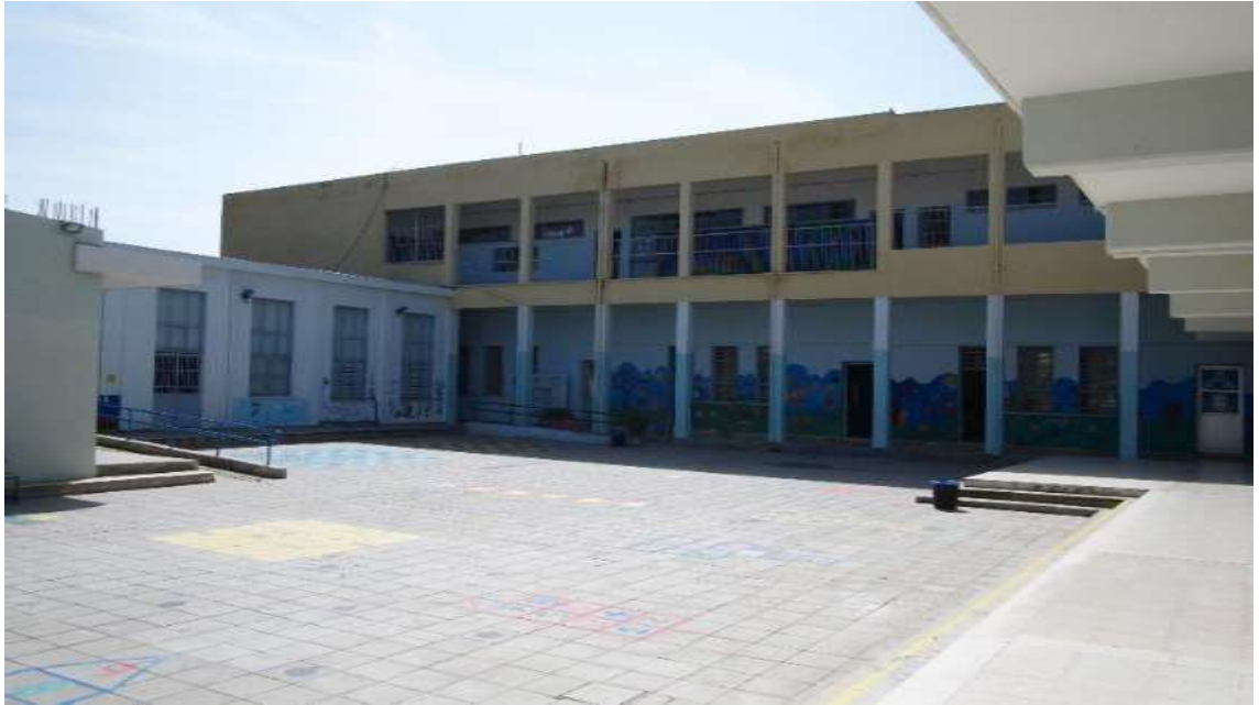
Il. 4- 24/AIES North façade of the school @ Author, March 2018
