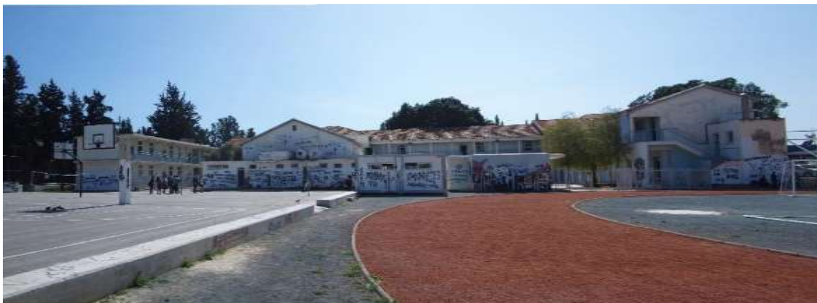
Il. 4- 24/DMS Northeast façade of the school @ Author, March 2018
