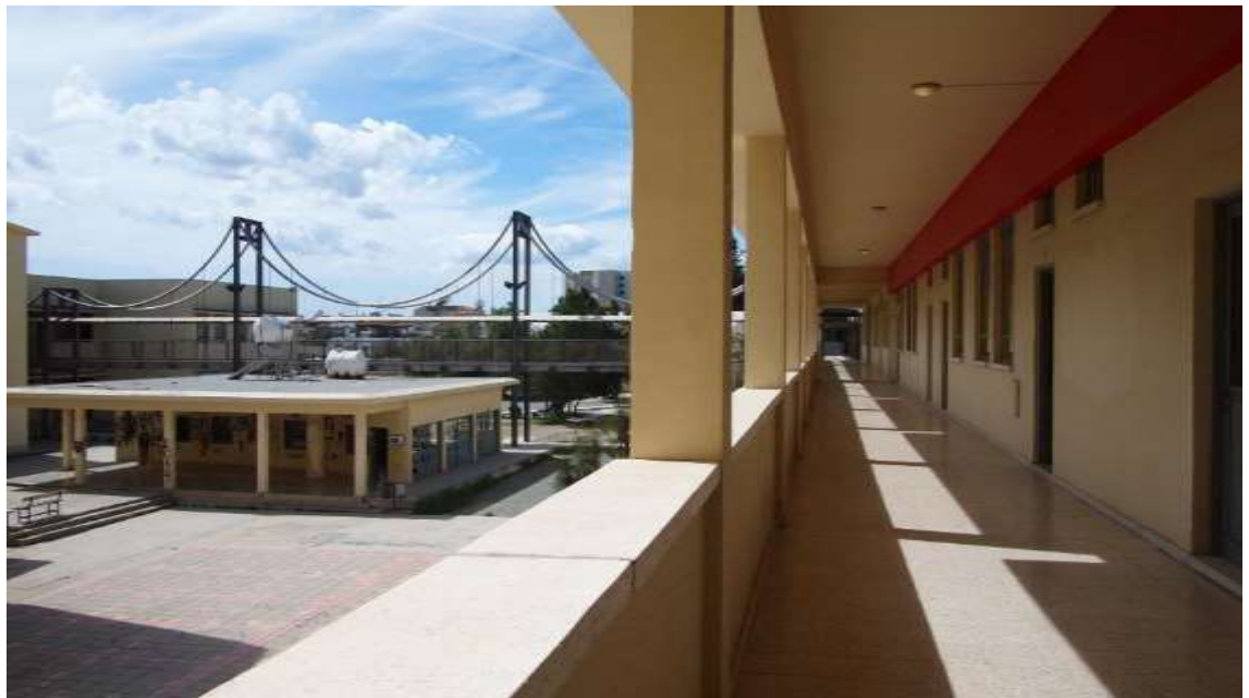
Il. 4- 28/AGHS View from the balcony of the north wing towards the school yard, view towards the west @ Author, March 2018
