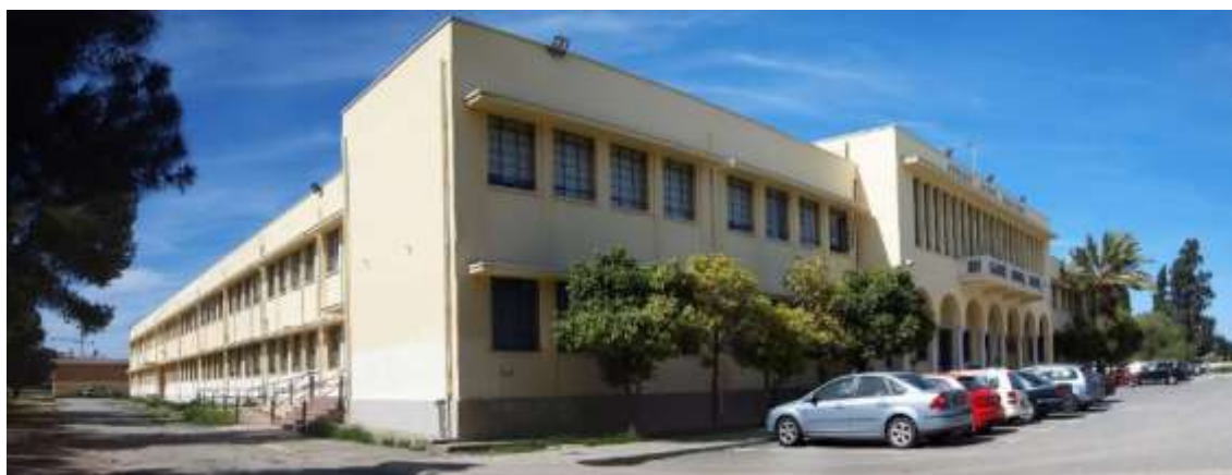
Il. 4- 12/AGES The southeast corner of the school's initial building, view towards the west @ Author, March 2018
