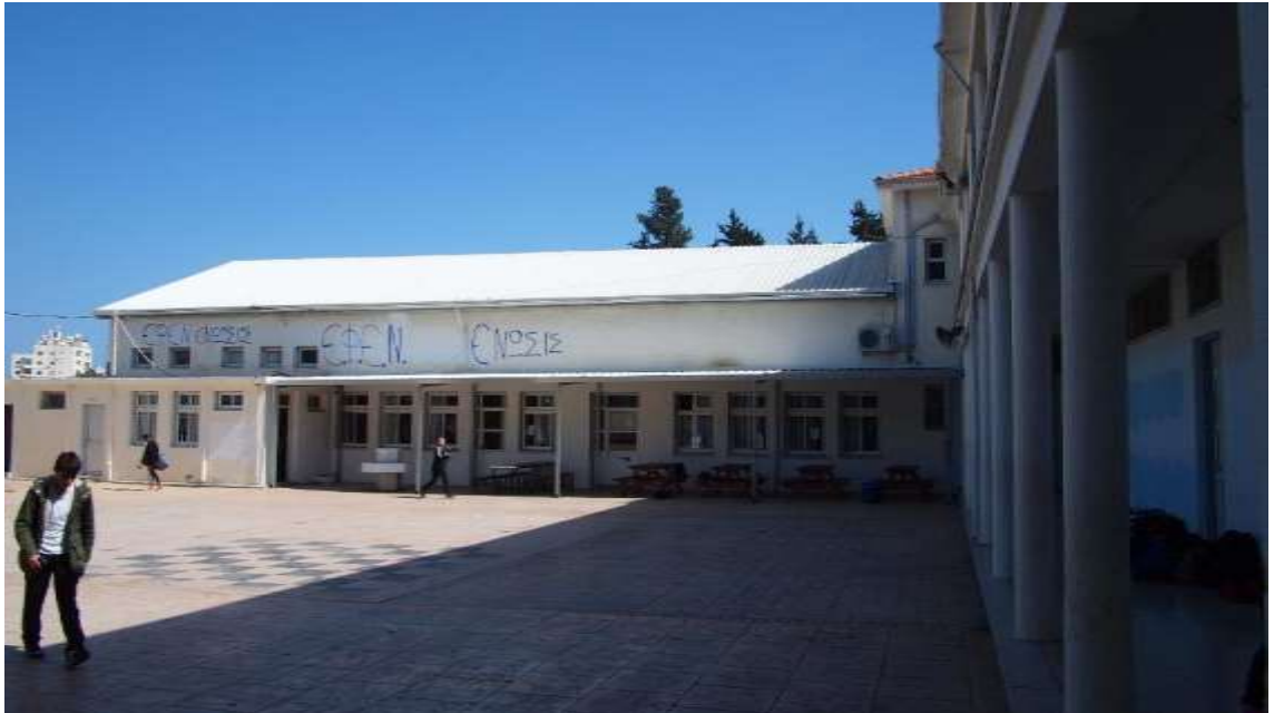
Il. 4- 28/DMS East façade of the school's more recent wing (east wing) @ Author, March 2018
