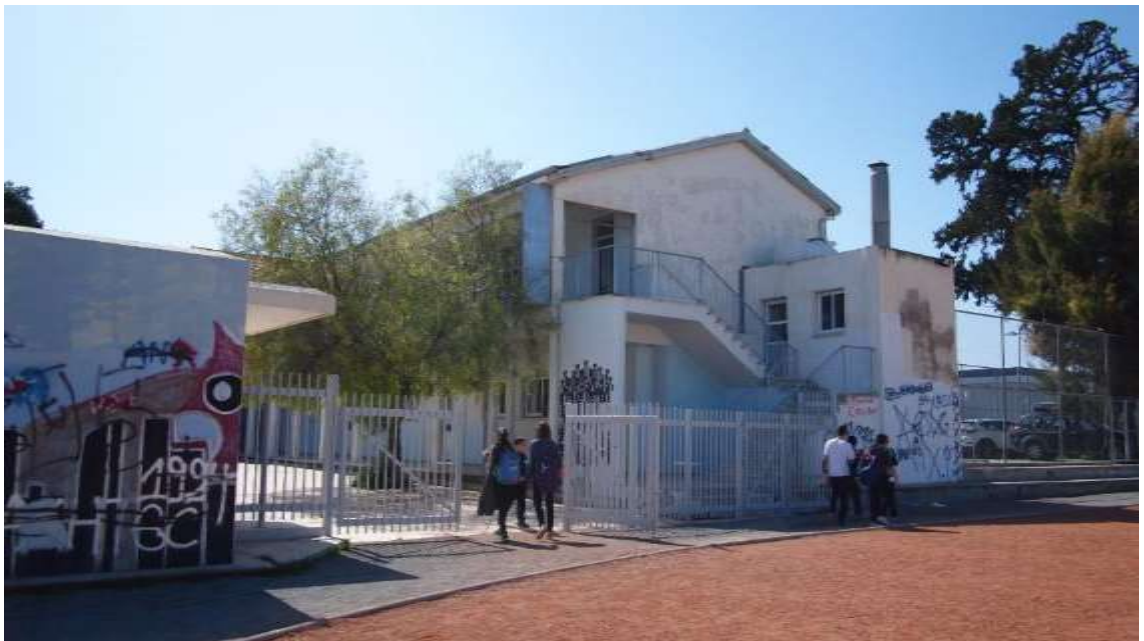
Il. 4- 23/DMS Northeast façade of the school @ Author, March 2018
