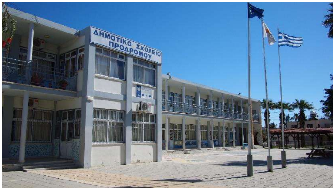
Il. 4- 22/PES Southwest façade of the school, view towards the northeast @ Author, April 2018
