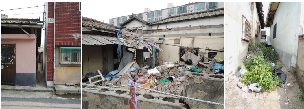
Figure 2-3. (1) A block with a very narrow entranceway where vacant houses are located inside; (2) a collapsed vacant house and piles of garbage dumped inside; and (3) a weedy, litter-strewn street around vacant houses
