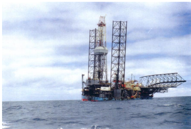
Fig. 2 Maersk Victory : punch-through failure (Aust, 1997)
