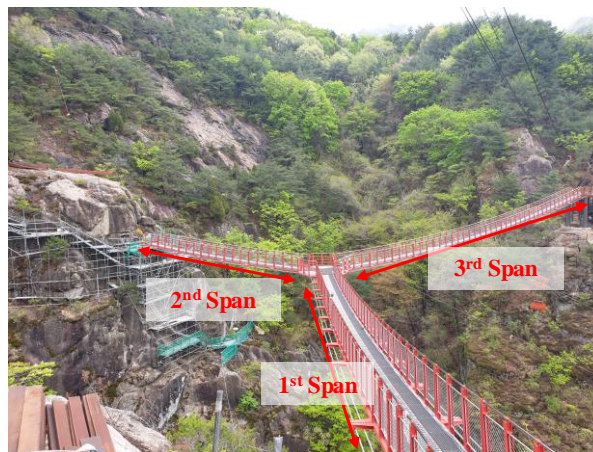
Fig. 3. 7. Geo-change suspended footbridge
