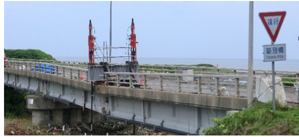
(b) Loading jack for static loading test Figure 1: Target bridge.
