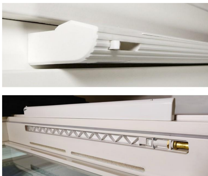
Figure 5. The trickle vent, Biobe ThermoMax A, used in the supply air windows of this study.
