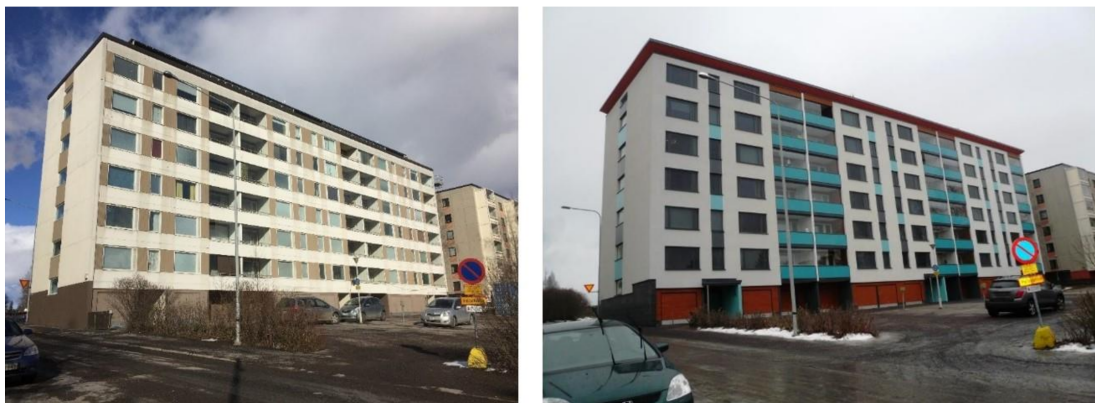
Figure 4. The studied building before and after retrofitting.
