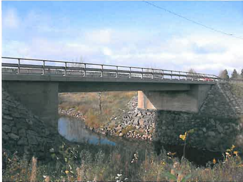
Figure 6.1. Jylhänranta concrete bridge in the middle part of Finland in Pulkkila.
