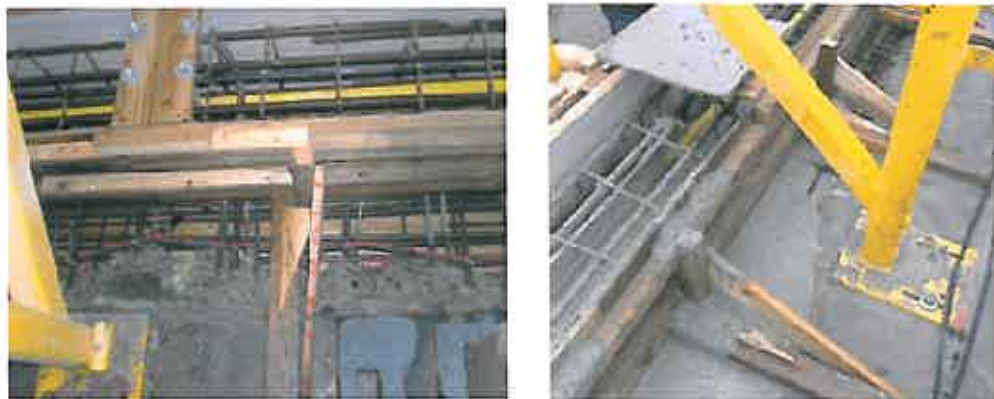
Figure 4.1.2. Two fibre optic temperature and moisture content sensors (red and black cables), VK1E1 and VK2E1, installed close to the joint area of the new and old part of the bridge.
