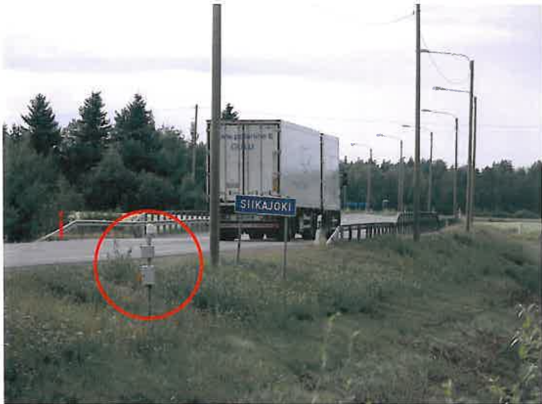
Figure 6.3.2. WSP's prototype of automation based monitoring system (circled) on the Jylhäranta Bridge.
