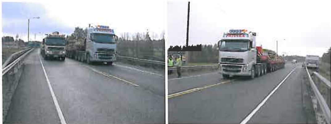
Figure 10.1.2. The heavy lorry and carriage used in the loading test in Jylhänranta bridge in 2007.
