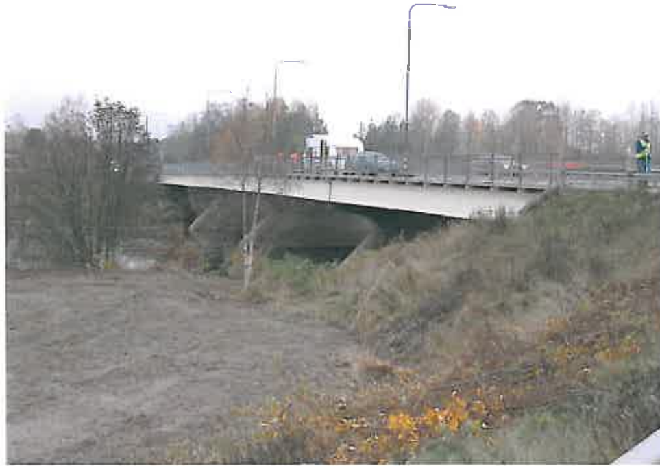
Figure 7.1. Siikajoki concrete bridge in the middle part of Finland in Revonlahti.
