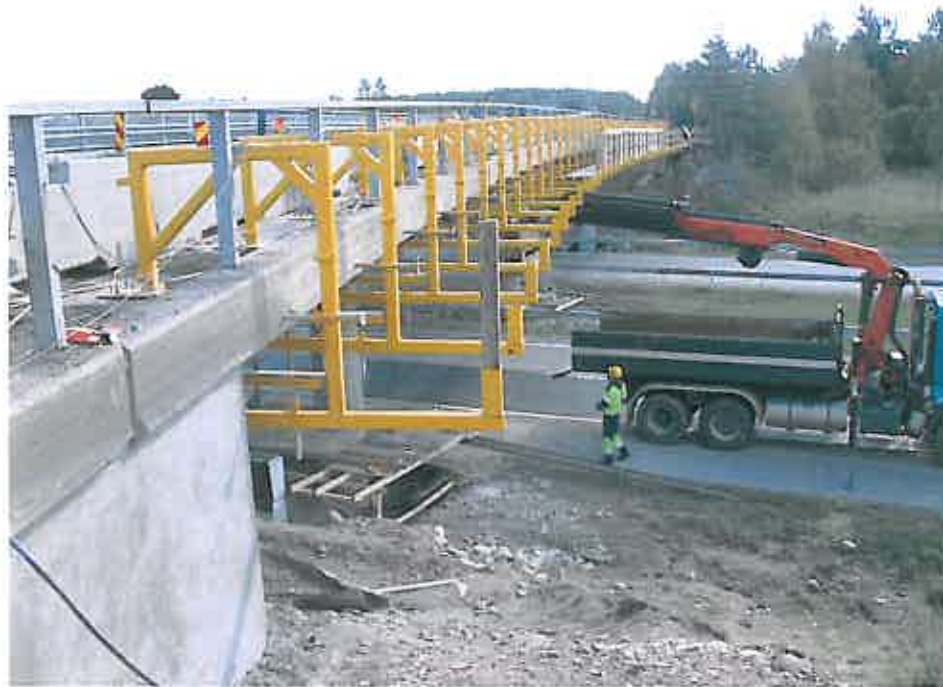
Figure 4.1. Boxby concrete bridge in Sipoo during rehabilitation.
