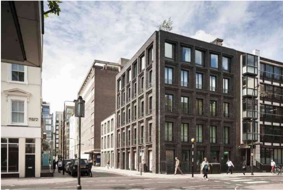
Facha principal de Corner House.
