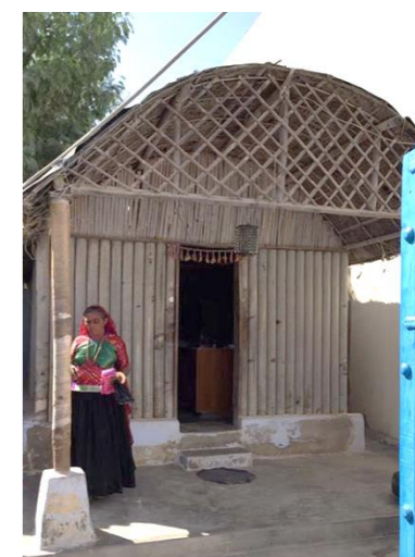
Fig 65. Paper Log House, India. Shigeru Ban, 2001.
