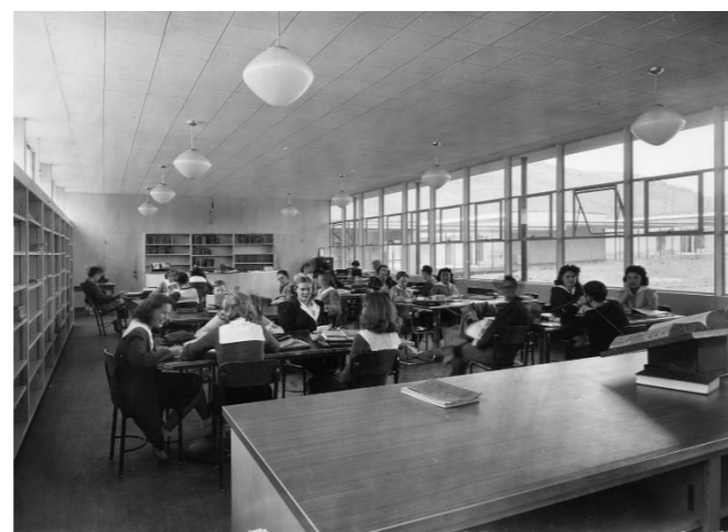
Espacio interior de Acalanes Union High School (1939) Erneste J. Kump.
