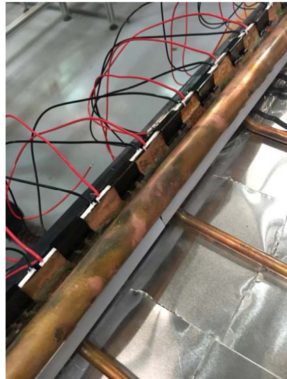
Fig. 4: Detail of the TEG and clamps installation
