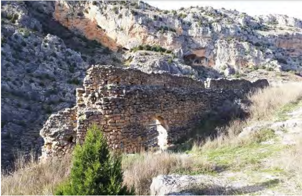
Figure 4. View of the wicket gate from the interior of the fortified precinct (J. Díaz).
