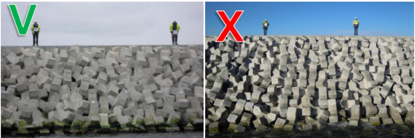
Fig. 2. Xbloc Armour unit placed with random orientation (left) & uniformly (right)
