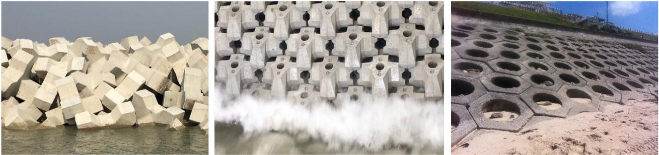
Fig. 1. Xbloc (left): Random placed interlocking, XblocPlus (middle): Uniformly placed interlocking, Seabee (right): Uniformly placed friction
