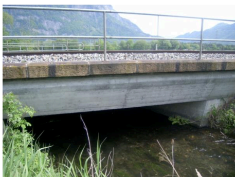
Fig. 8: Culvert through the railway dike [6]
