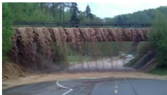
Fig. 1: Flood overflow from and discharge under a road bridge [1]
