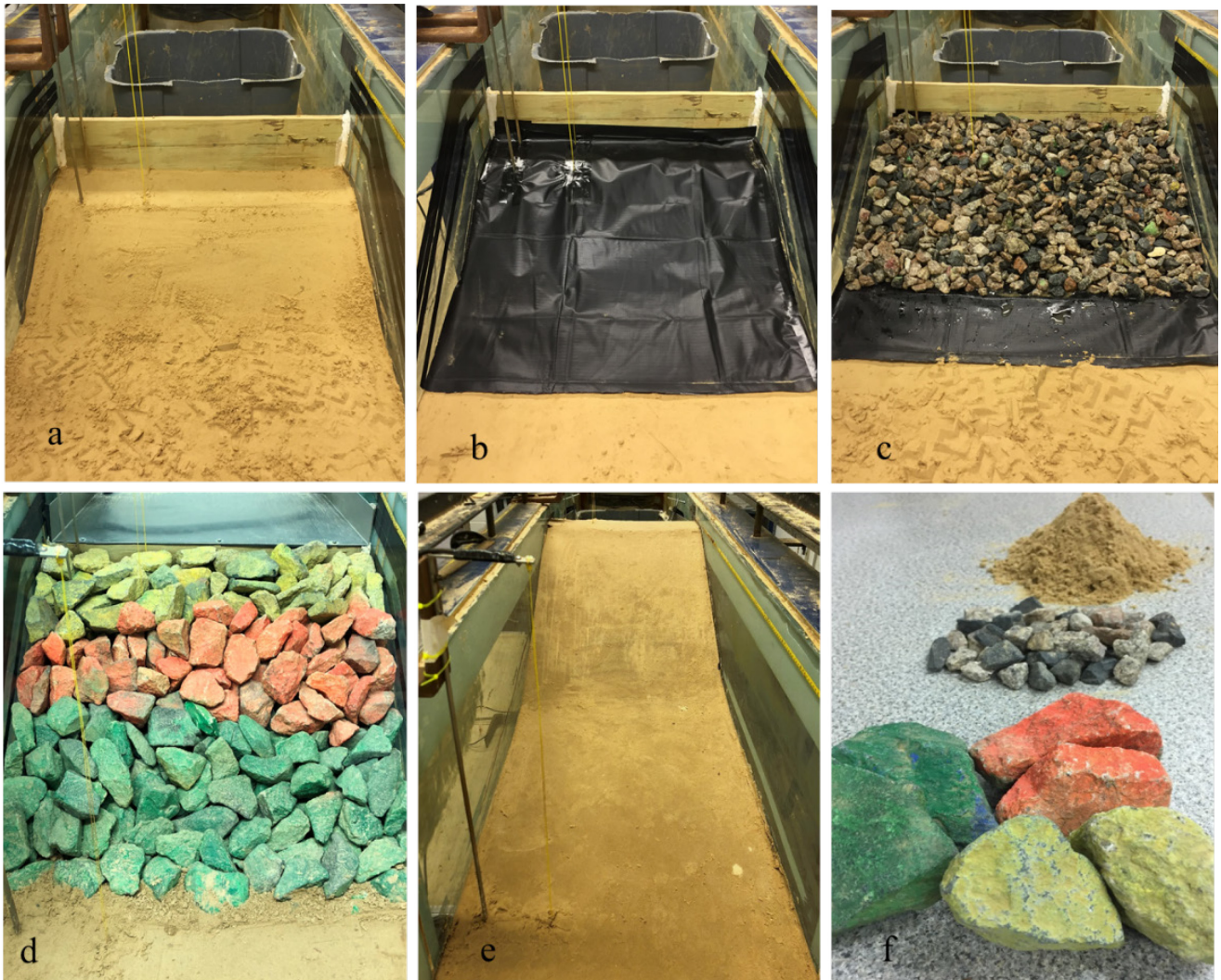
Fig. 2. Photos detailing the hybrid structure construction procedure. The sandy core of the rubble mound fronting the vertical wall (a) was covered by a geotextile fabric (b) to prevent the movement of sediment underneath the rocks. Gravel with a nominal diameter of 2 cm was used to construct the filter layer (c). Rubble mound structure before applying the sand cover (d). Finished hybrid coastal structure with sand cover of 9 cm thickness before the first wave run (e). Used materials are shown in Panel f. (Almarshed, 2019)
