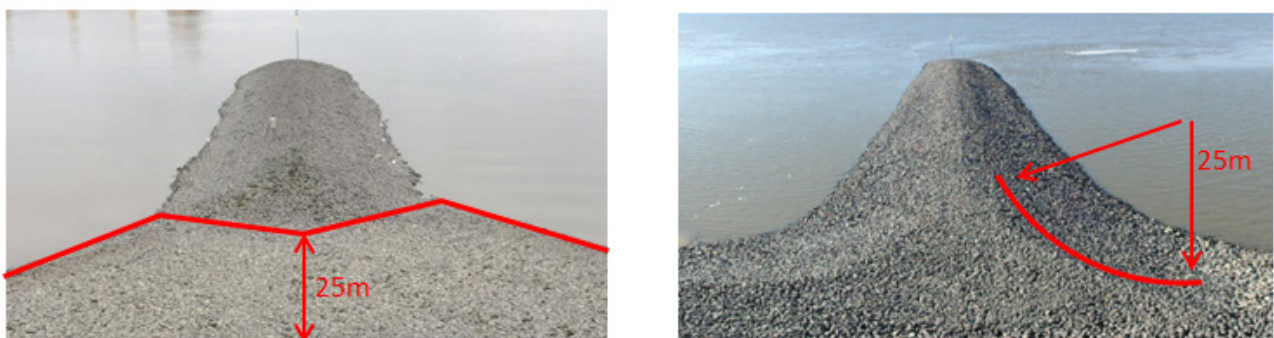
Fig. 5. Optimised groyne root designs: recessed groyne B29 (left), large-radius groyne root B31 (right).
