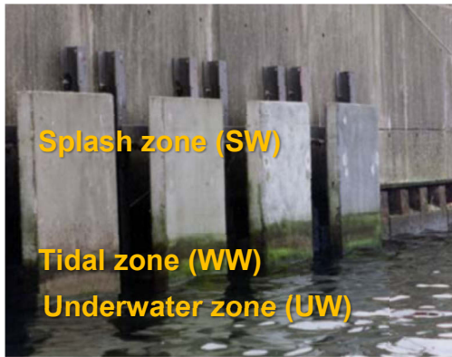
Fig. B.5: Exposed slabs on the Baltic Sea coast
