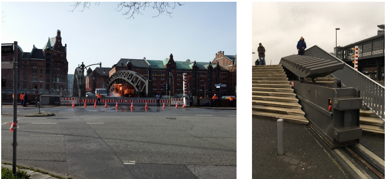
Fig. 4. Left: regular semi-annual testing of gate 'Brooksbrücke' in Hamburg (courtesy TUHH). Right: Low-effort partial testing of gate 'Niederbaumbrücke' in Hamburg (courtesy TUHH).
