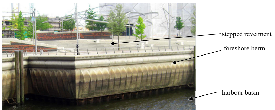
Fig. 1. Impression of the Marco Polo Terraces with dominant foreshore berm and adjacent stepped revetment located at a former harbor basin in Hamburg, Germany (view from offshore the harbor basin).
