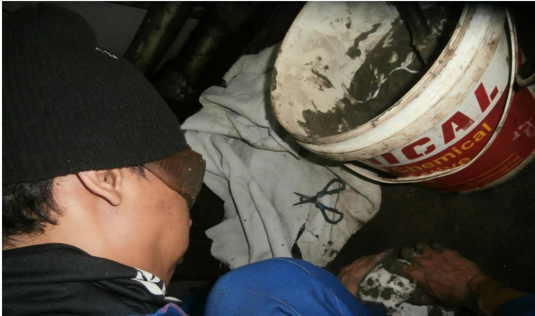
Gambar lampiran 1 : proses plugging economizer tube
