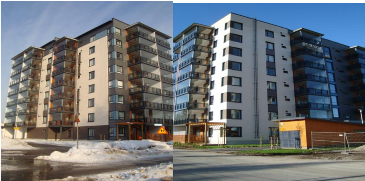
Figure 6. Block houses in Suvilahti Vaasa use geothermal and solar energy. [9]
