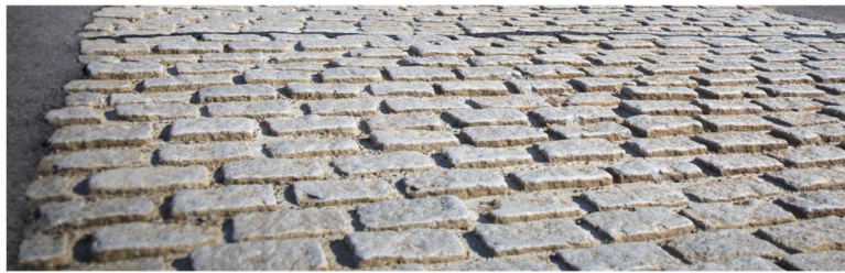
Figure 5: Belgian pave road surface [15].
