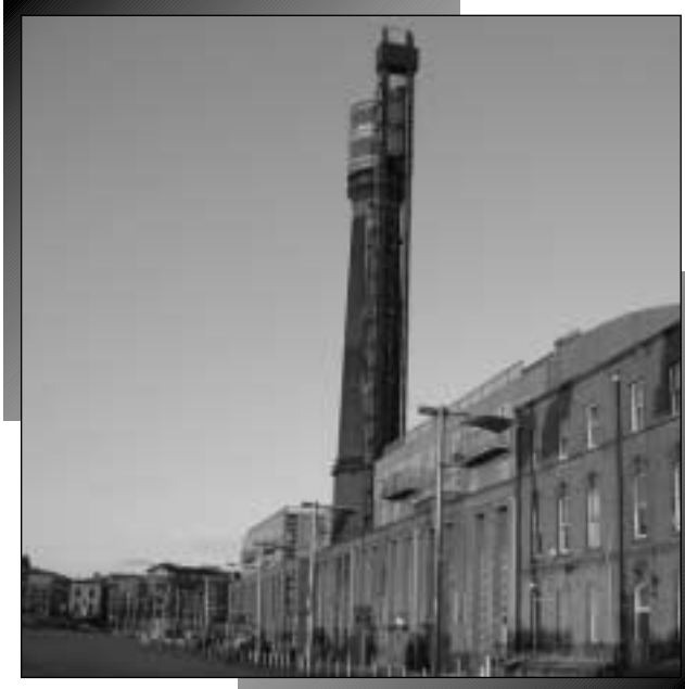
► Chimney Viewing Tower, Smithfield.
