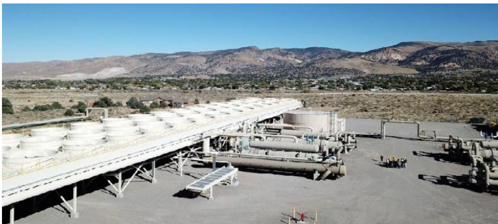
Figure 9. Binary cycle geothermal power plant in Nevada, USA [11]
