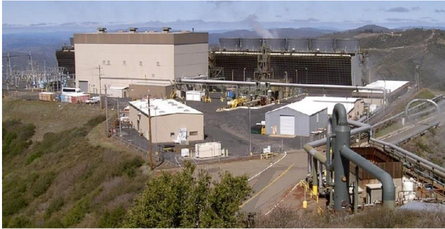
Figure 5. Dry steam geothermal power plant, The Geysers, California, USA [11]
