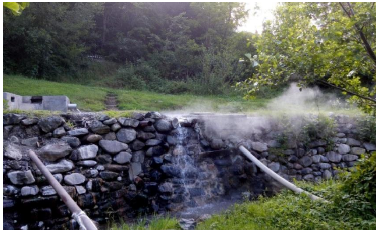
Figure 2. Hot water flowing artesian well in Jošanička Banja spa of temperature of 78 °C [6].
