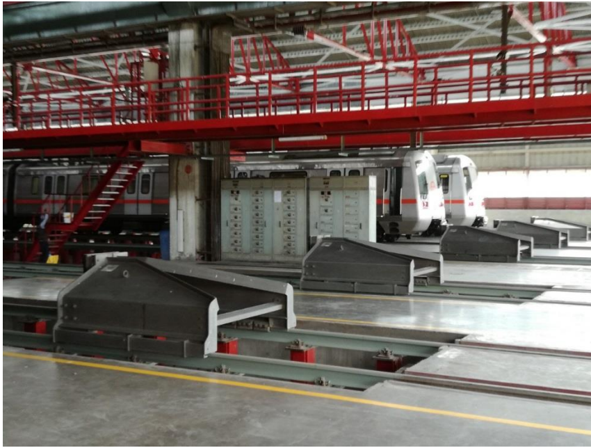
Figure 4.5: The Sharsti Park Depot inside DMRA
