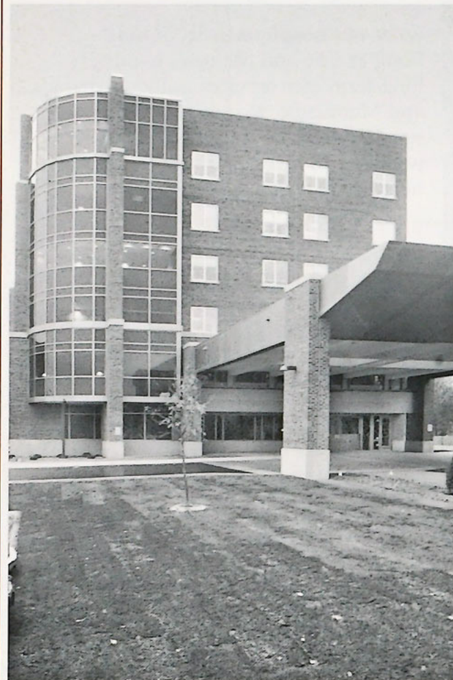
St. Cloud Hospital northwest addition
